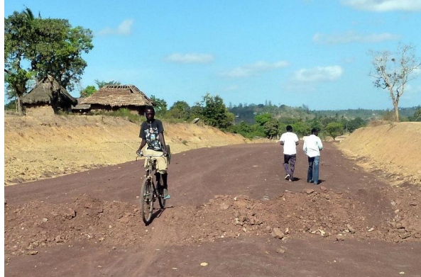
Road under construction at Giriama, Kenya
