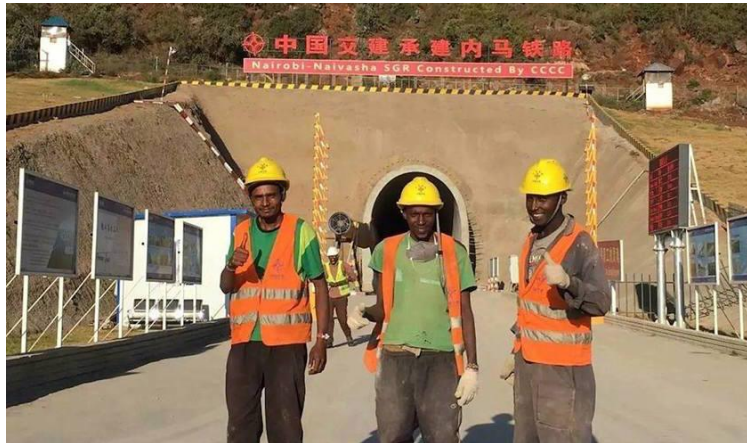
Workers at a new tunnel on the Nairobi-Navaisha standard gauge railway (SGR) project in Kenya
