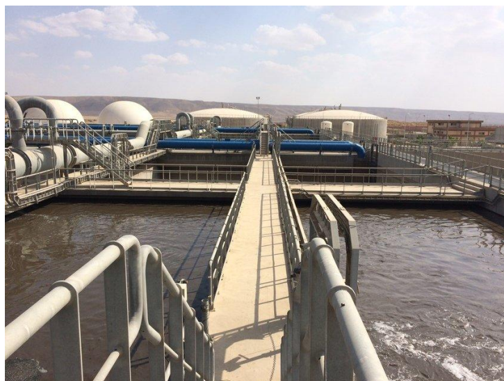
The New Cairo wastewater treatment plant built and operated by FCC Aqualia
