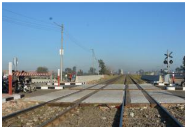
Egyptian government focuses on upgrading its railway infrastructure.
